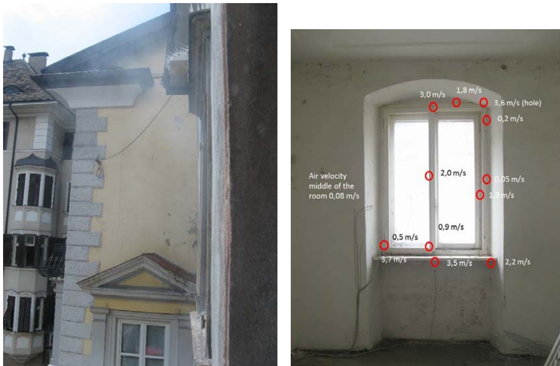
Figure 2 and Figure 1: Gas through the windows, air velocity near the window
