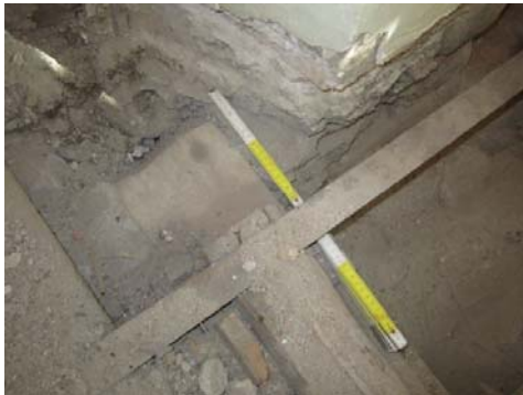
Figure 9: Opening of wooden beam ends
