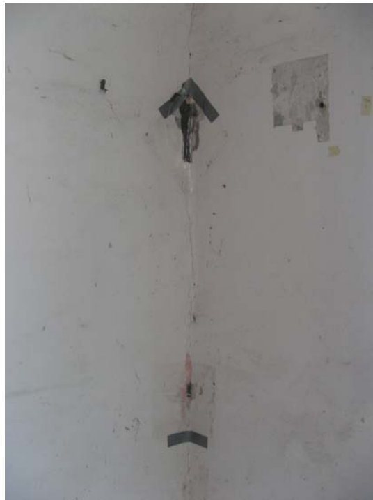
Figure 3: Sealed cracks on the interior wall
