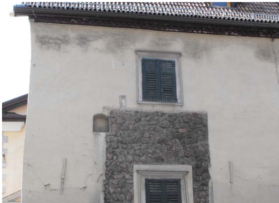
Figure 4: Eastern façade: additional information on masonry structure also behind plastered areas
