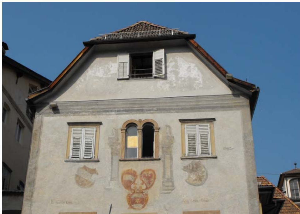
Figure 6: Southern façade: information on masonry structure in plastered areas, arc construction, attic
