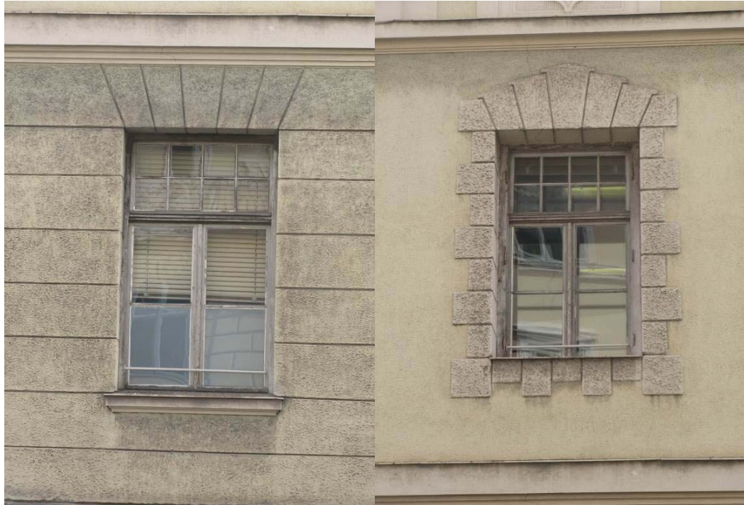
Figure 4.19: Box-type window of the “Aufschnaiter Middle School” in Bolzano
