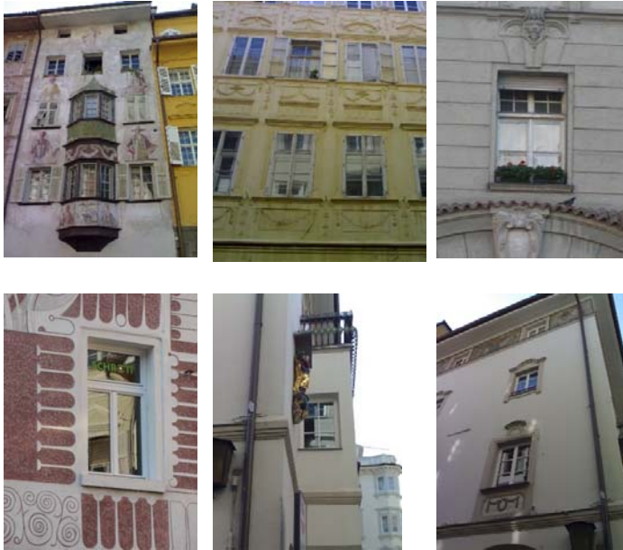
Figure 30-35: Originally, the wooden frames, impost and sash bars were very fragile and thin, possibly moulded (fig. 30-32), while the optic of the typical replacements is much broader (simple application of the IV68 standard, fig.33-35).
