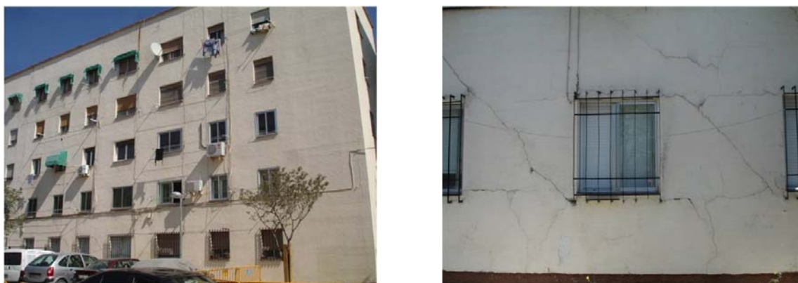
Figure 2 – South facing façade
