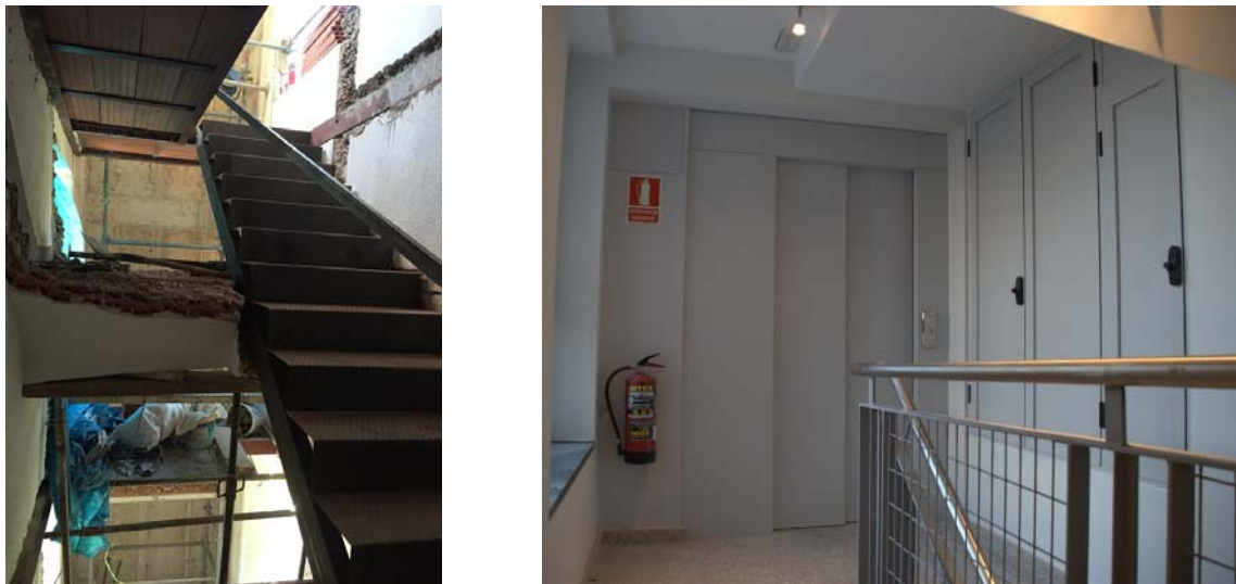
Figure 22 – Newly setup staircase during and after installation completion
