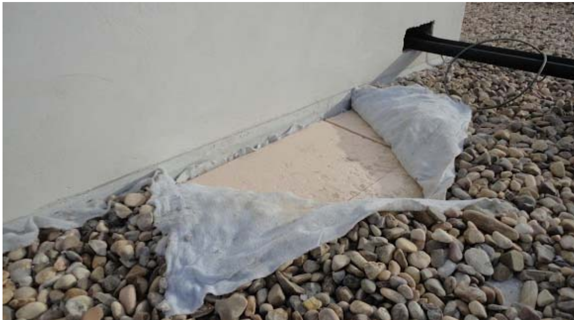
Figure 26 – XPS roof insulation
