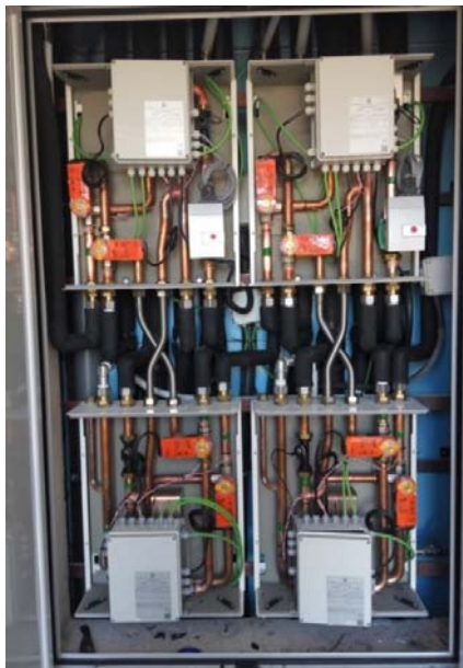
Figure 37 – Energy Hubs connections
