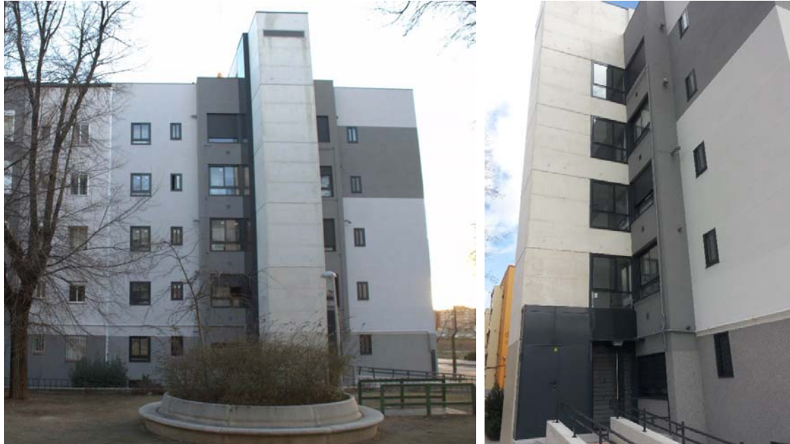
Figure 27 – North façade after retrofit
