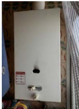
Figure 13 - Gas boiler
