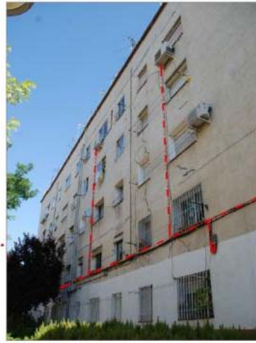
Figure 7 - Telephone lines
