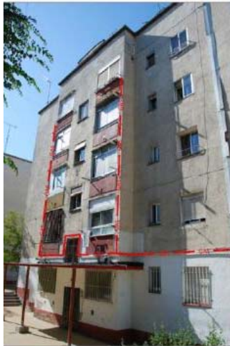
Figure 6 - Gas piping
