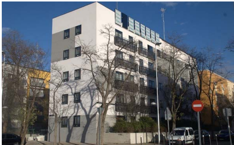
Figure 30 – South-facing façade with solar collectors installed
