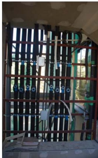
Figure 36 - Vertical pipelines construction
