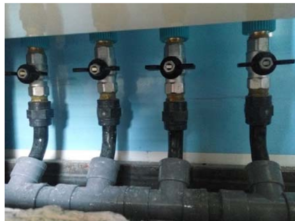
Figure 38 Safety door on the hallway and emptying system of the verticals lines
