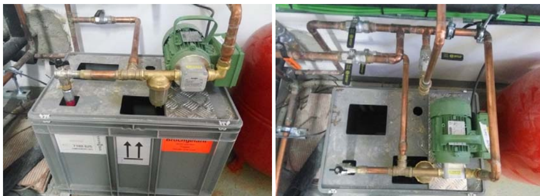
Figure 34 - Mixing system
