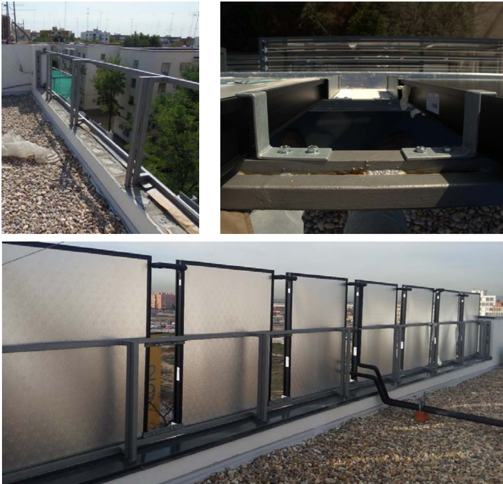
Figure 29 – Solar field installation on the south facing parapet
