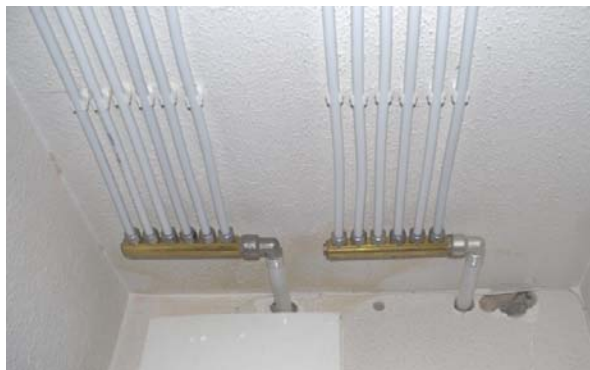
Figure 40 - Piping distribution in the corridor of the dwellings
