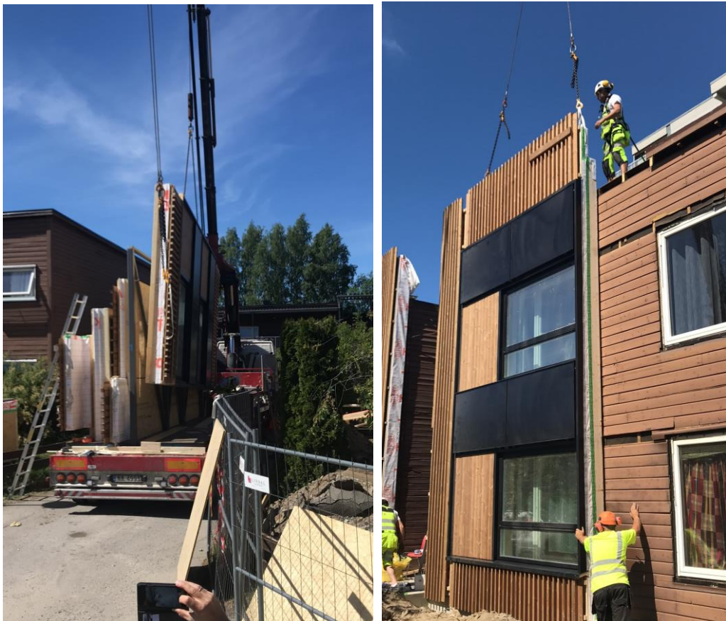
Figure 28: Safe craning and careful securing of element, right on spot without tolerance problems
