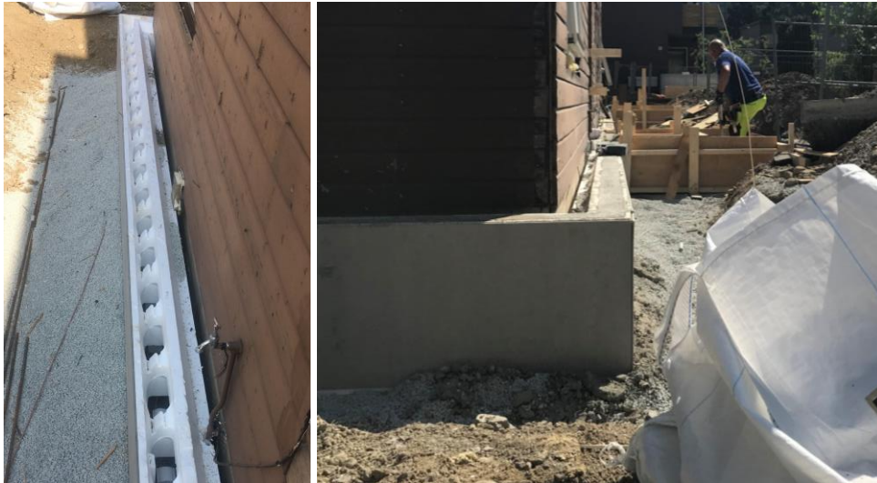
Figure 26: Foundation molds before casting (left) and after filling of concrete (right)
