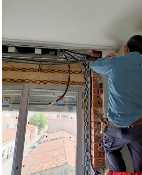
Figure 119 (left) PMF Façade panels anchored. (right) Inside finishing works
