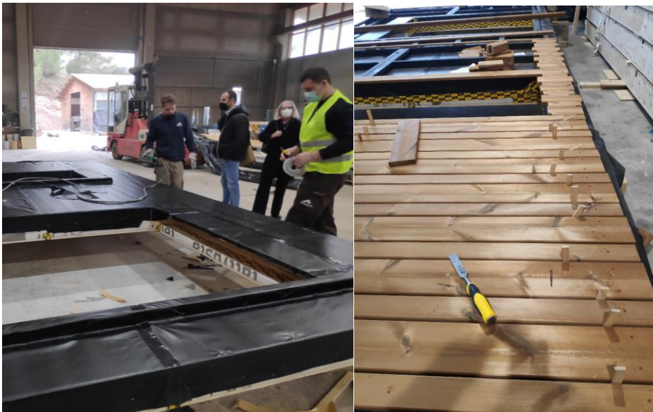
Figure 114 Picture (left) waterproof layer installation. Picture (right) Mounting external cladding
