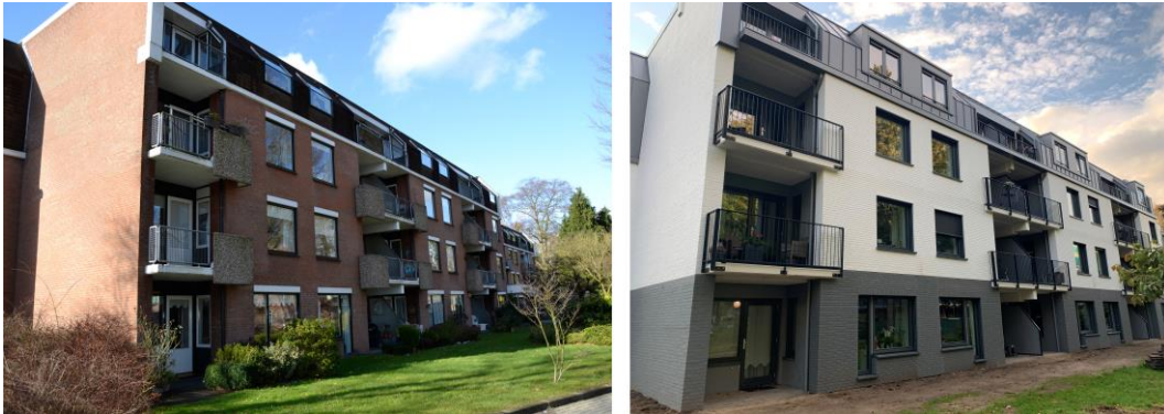
Figure 52 Marienheugel before and after renovation
