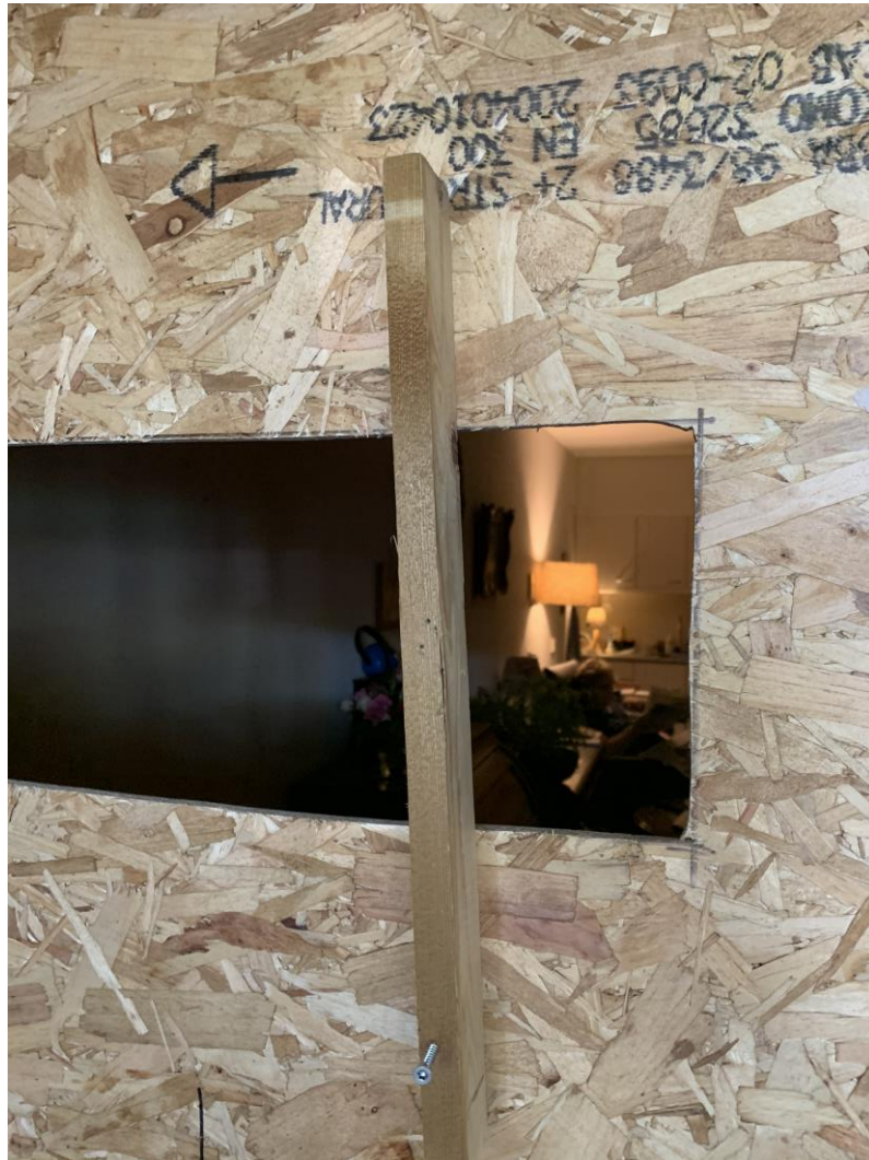
Figure 68 Very small daylight opening in the temporary wall.
