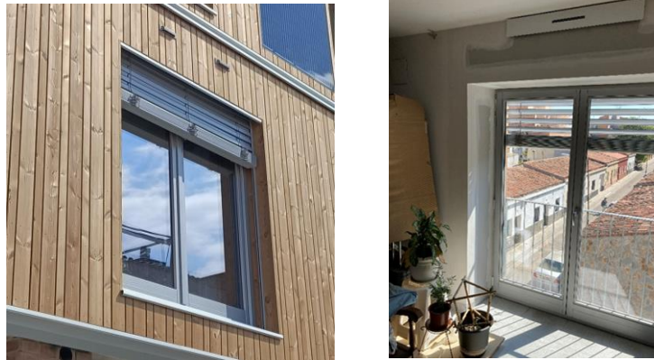
Figure 92. New aluminum folding shutter compatible with ventilation ducts
