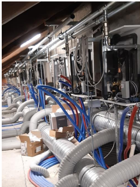
Figure 136 NRGate Box™ settled and to be connected during installation
