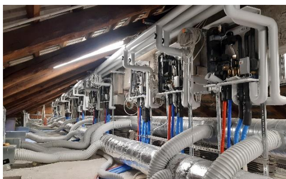
Figure 4 Italian Demo renovated building
