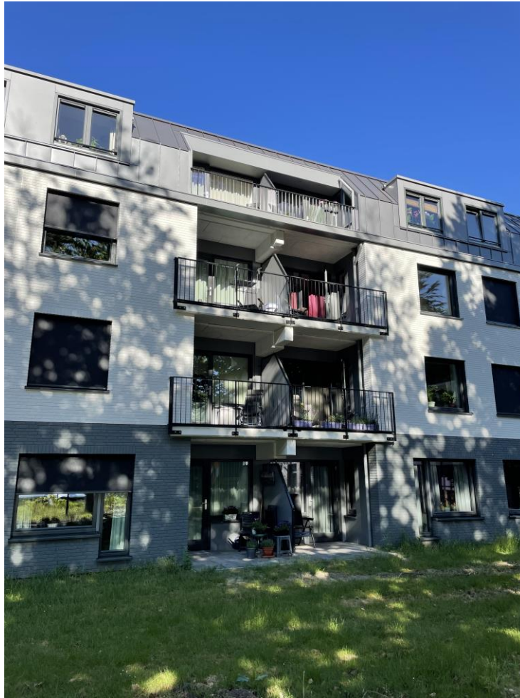
Figure 60 Façade of the 4RinEU demo part: new prefab façade with new triple glazed windows, integrated shading and thermal bridge insulation around the balcony
