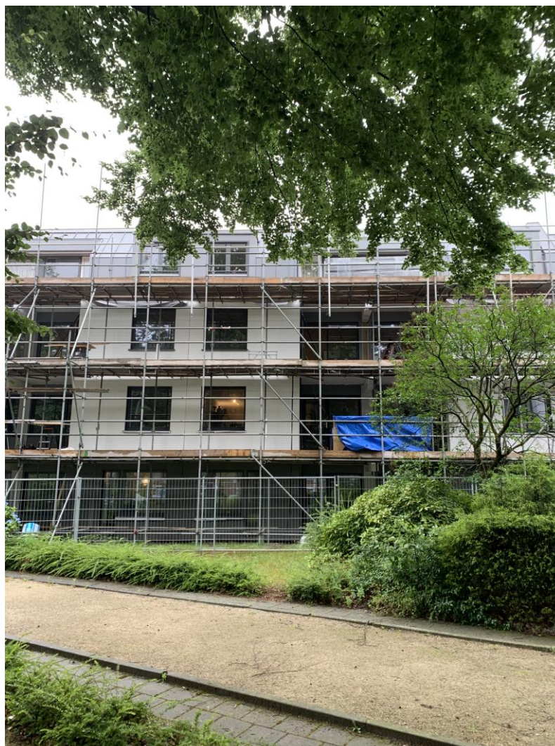
Figure 70 Mounted prefabricated façade elements after a two-weeks period for all 15 apartments.
