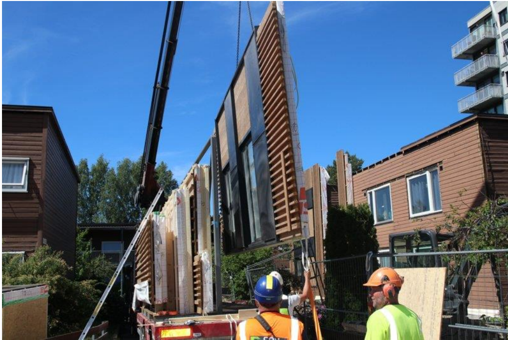
Figure 27: installation of south façade elements with PV
