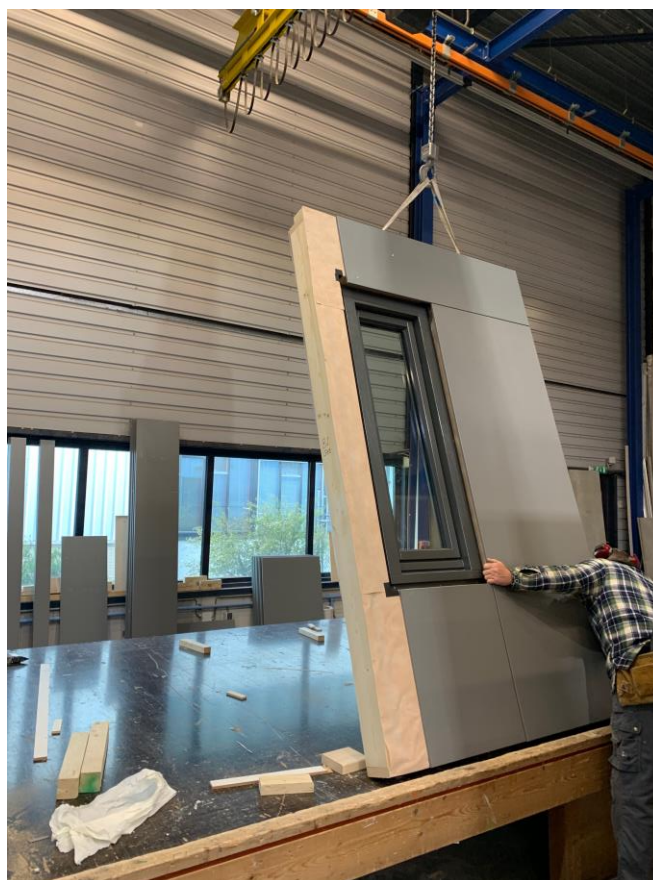
Figure 63 Window frames and glazing were pre-installed in the factory.
