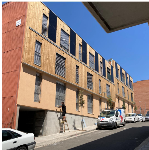
Figure 3 Spanish Demo renovated building
