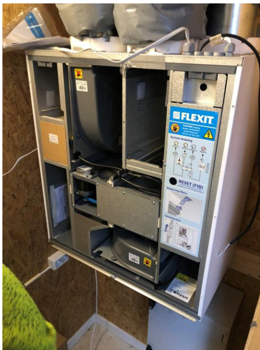
Figure 17 Air Handling Unit (AHU) Flexit Uni 3
