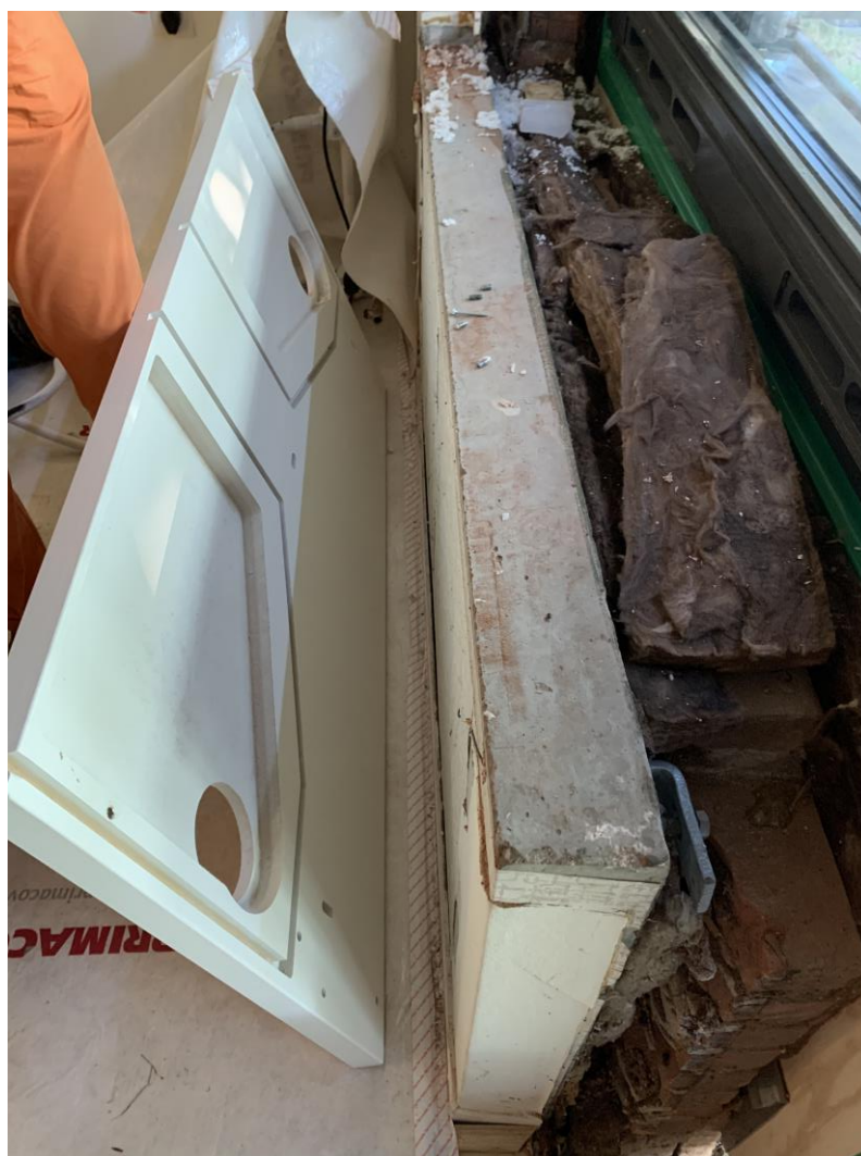
Figure 80 Specific timber device which guides fresh air from the façade into the decentralized ventilation unit.
