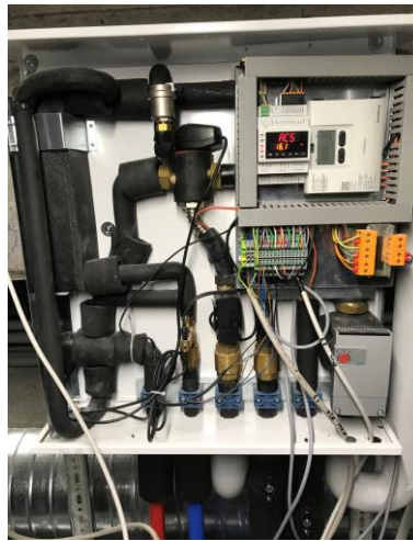
Figure 135 Inside the NRGate Box™ during installation
