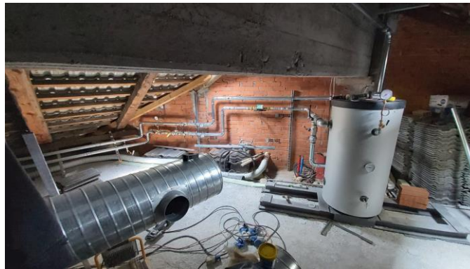
Figure 139 Hydraulic system during installation
