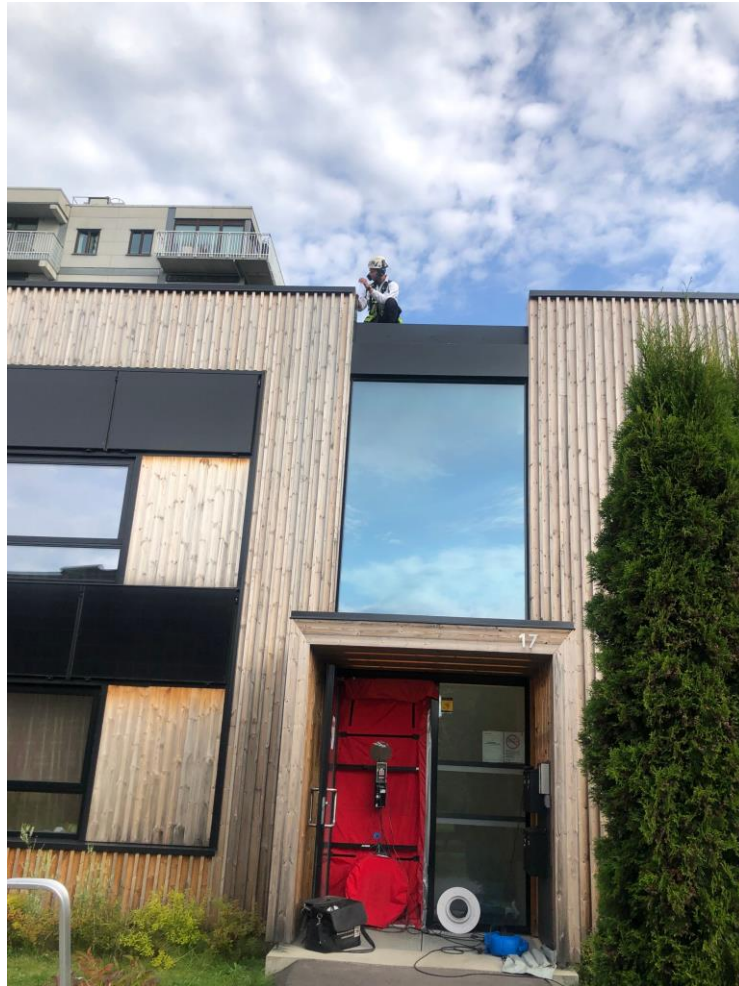
Figure 45: Blower door measurement performing while Lindal personnel is checking the sealing of the roof
