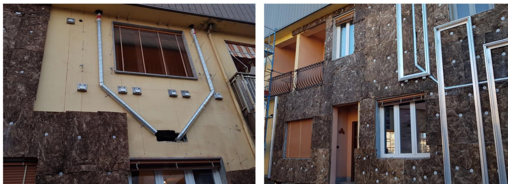
Figure 123 Installation of ventilated façade with ducts passage
