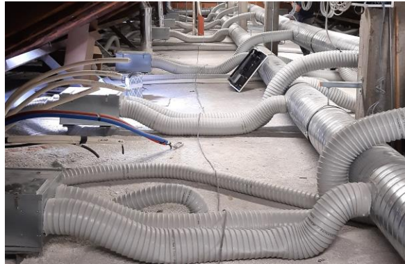
Figure 126 Ventilation ducts and recovery units during installation
