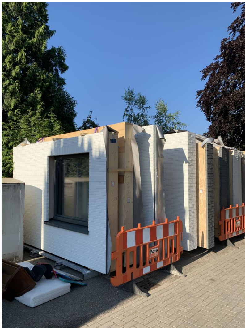
Figure 64 Prefabricated elements delivered to the site and waiting to be mounted
