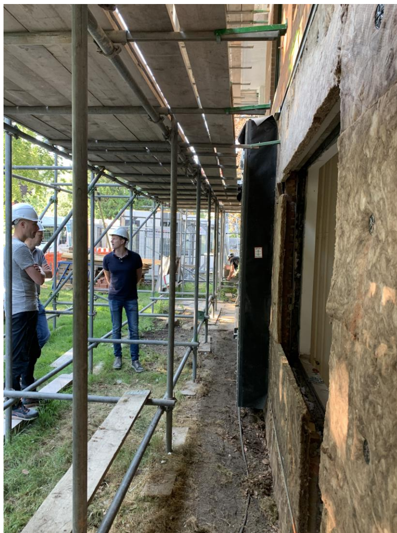
Figure 69 The prefab elements have been mounted horizontally. This reduces the disturbance and presence of construction workers. The original plan was to mount the elements vertically, which is easier from a technical perspective. The argument of tenants disturbance prevailed because of pandemic prevention measures.
