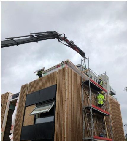
Figure 31: Mounting of the roof construction. Photo: Boligbygg
