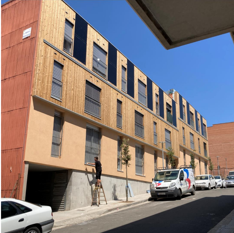
Figure 86: Spanish demo with the renovation almost finished.
