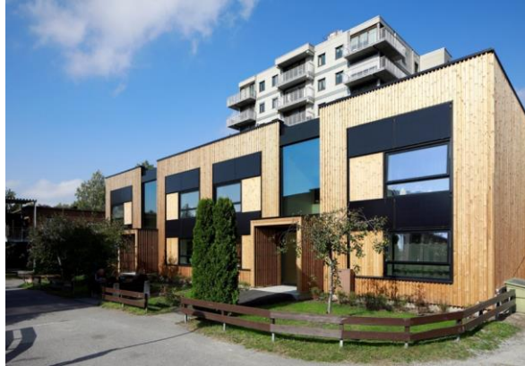
Figure 1 Norwegian Demo renovated building
