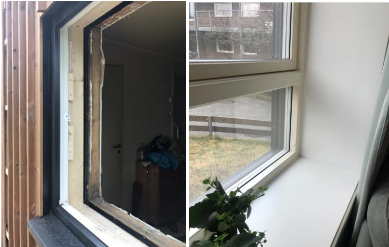
Figure 32: Installation of the windows in the prefabricated elements
