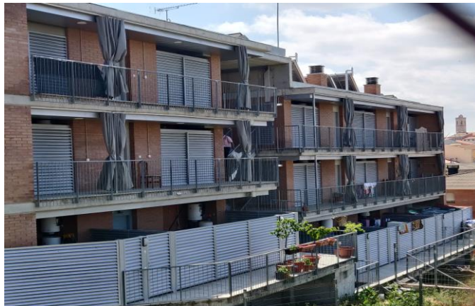
Figure 93. West facade with the sun protection curtains
