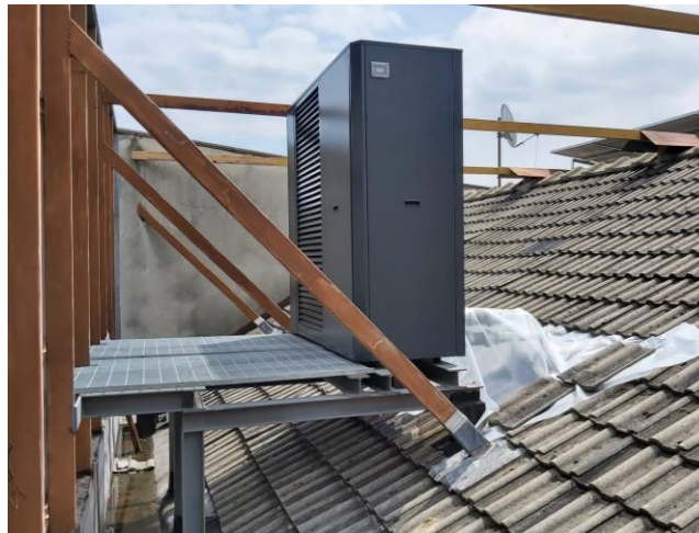
Figure 133 Heat Pump in Pinerolo during installation
