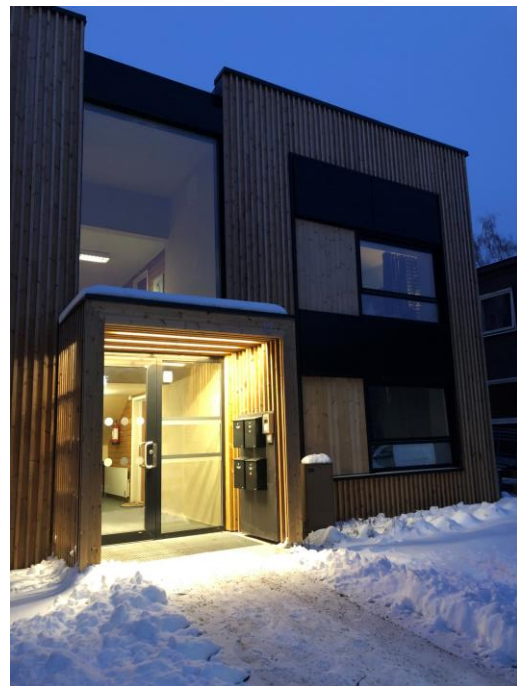
Figure 51: Haugerudsenteret in full operation after renovation, December 2018
