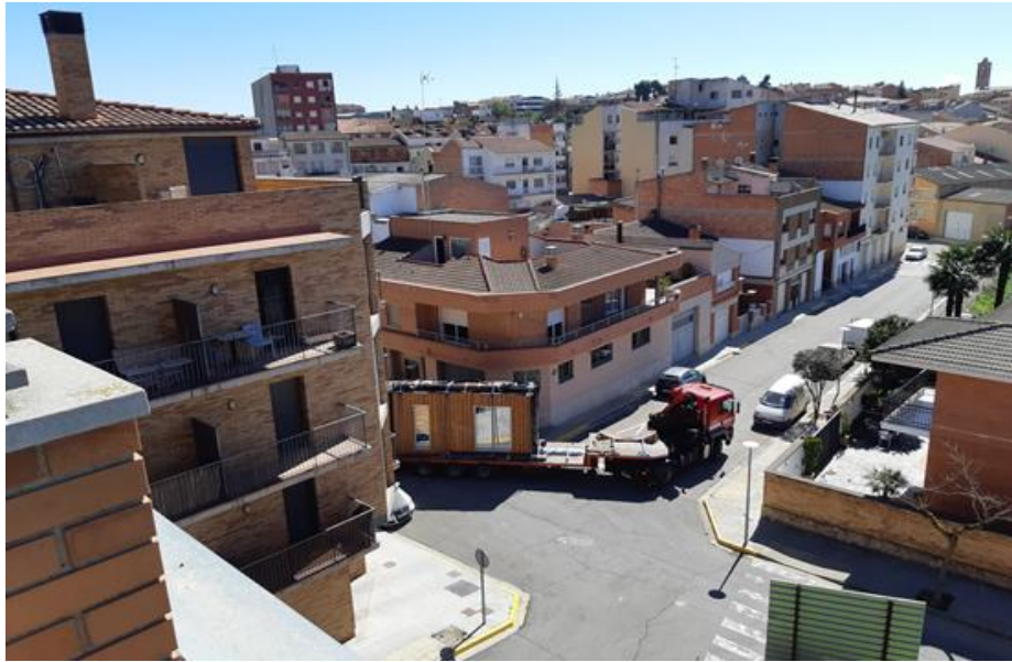
Figure 116 Arrival of the 1st PMF Façade panels to Bellpuig (date:18.03.2021)
