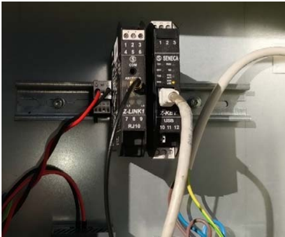
Figure 20 - Data reception from Transmitter (z_Link1) and Pyranometer (Z-KEY)
